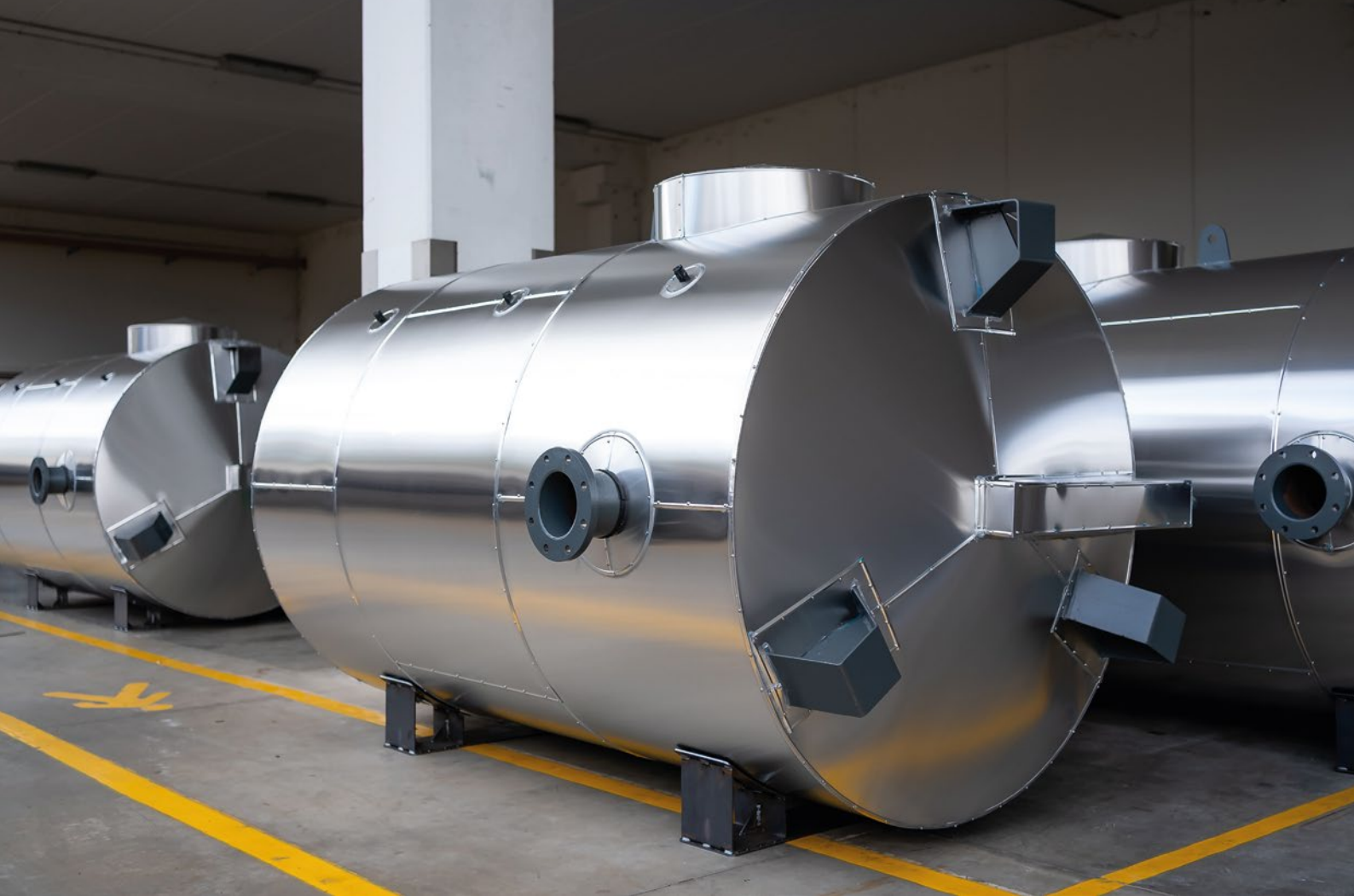
5.000 L chilled water buer storages for a datacenter in Amsterdam
